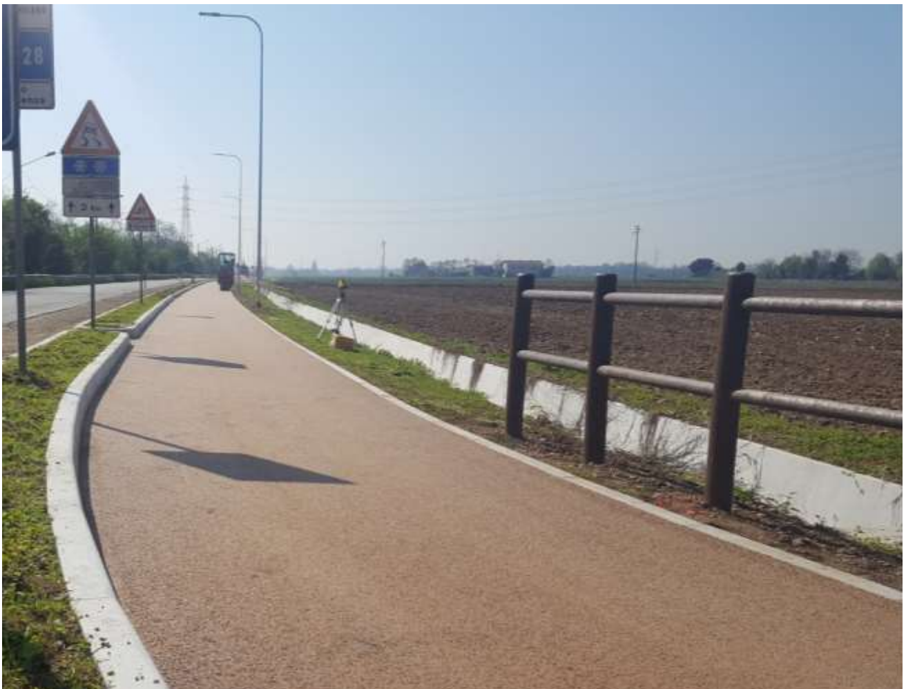
Paving laying around 2,000 sq - Thickness of 3 cm - Company RIMOLDI Cerro Maggiore MI
