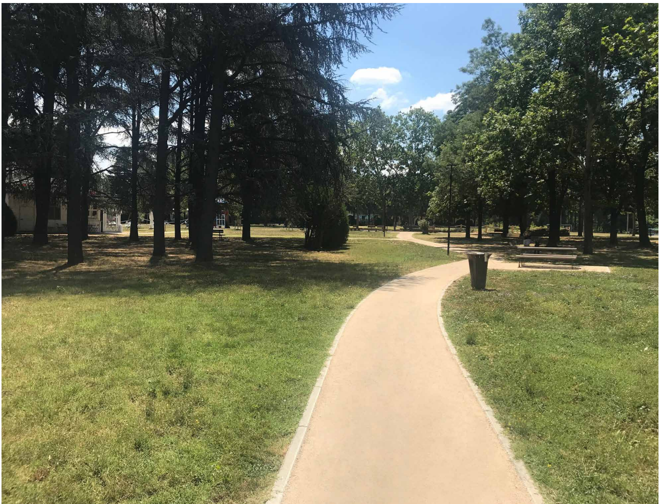
Paving laying around 1,000 sq - Thickness 4 cm - Company Marchesi Movimento Terra S.r.l. Pianoro BO
