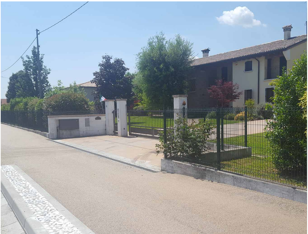
Paving laying around 2,000 sq - Thickness of 4 cm - Company DEON Belluno BL
