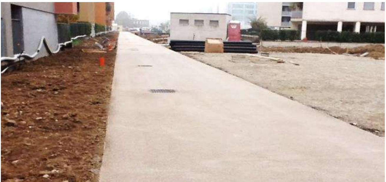
Paving laying around 3,000 sq - Thickness of 3 cm - Company UNISTRADe Monza MB
