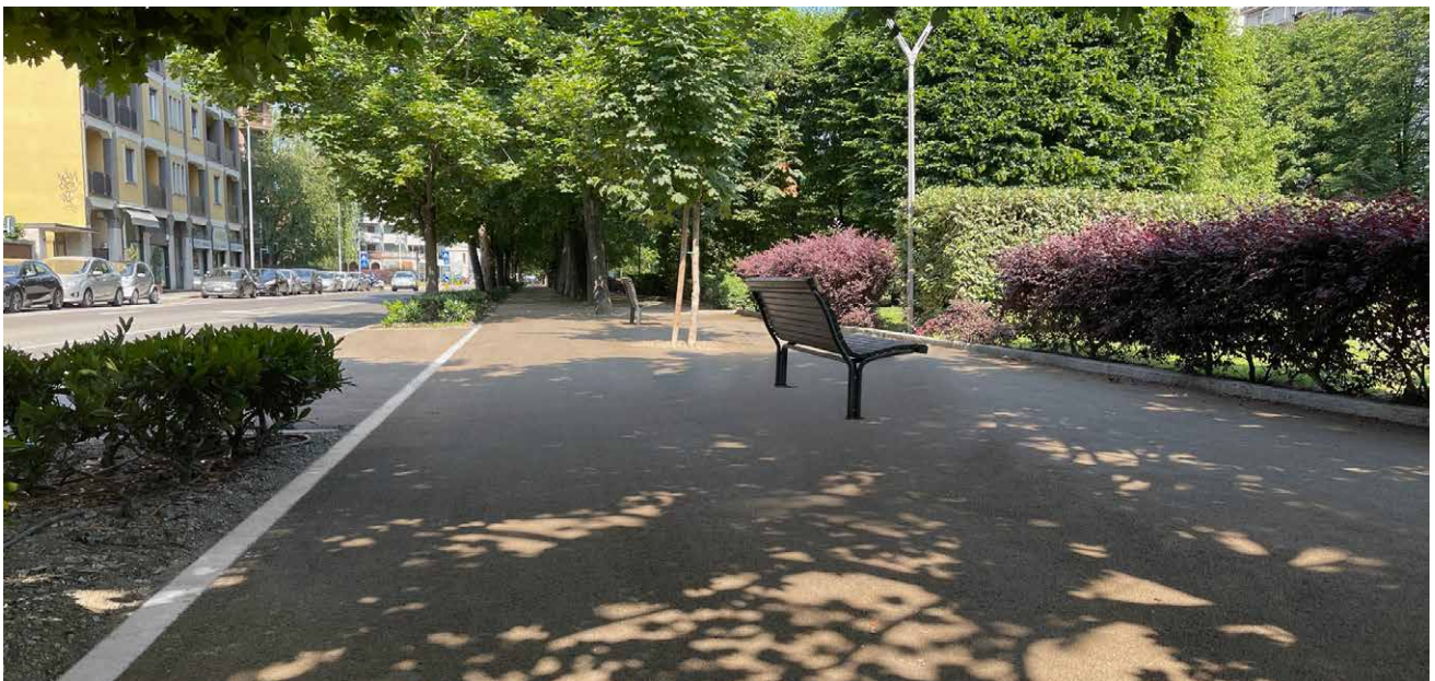
Paving laying around 1,400 sq - Thickness 3 cm - Company Kumar Snc - Villanova del Sillaro LO
