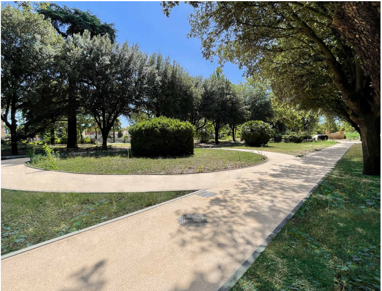
Paving laying around 1,800 sq - Thickness 3 cm - Company Sintexcal S.p.A. Ferrara FE
