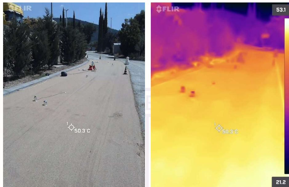
Figure 38. Test field and relative thermography.
