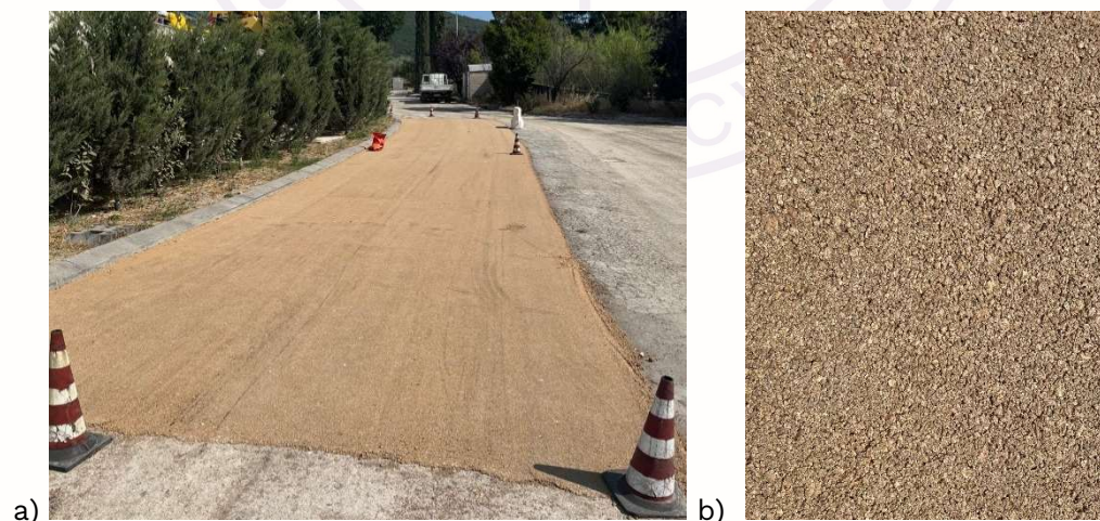
Figure 32. a) Test field, b) focus on the pavement.
